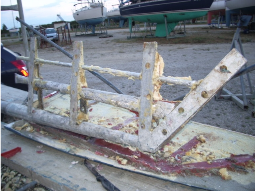
2 pics showing the separated alu frame/ shaft This had to be repaired by welding a smaller area
